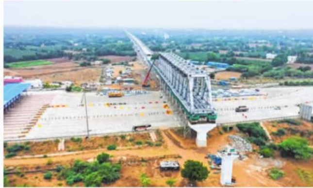
An aerial view of the newly installed structure
